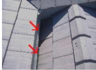
Although no sign of leakage is noted today, chance for water leakage is significant and will increase as the roof
